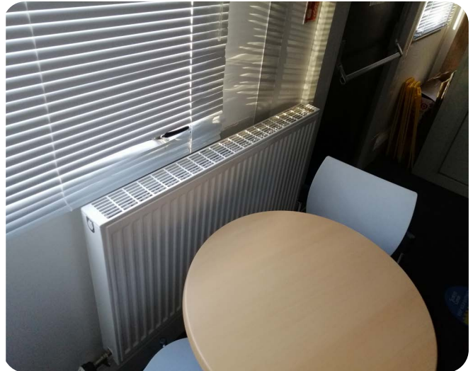
Mixed radiator types - - would need to be reviewed and upgraded for a heat pump system
