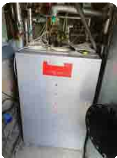
Decommissioned water source heat pump
